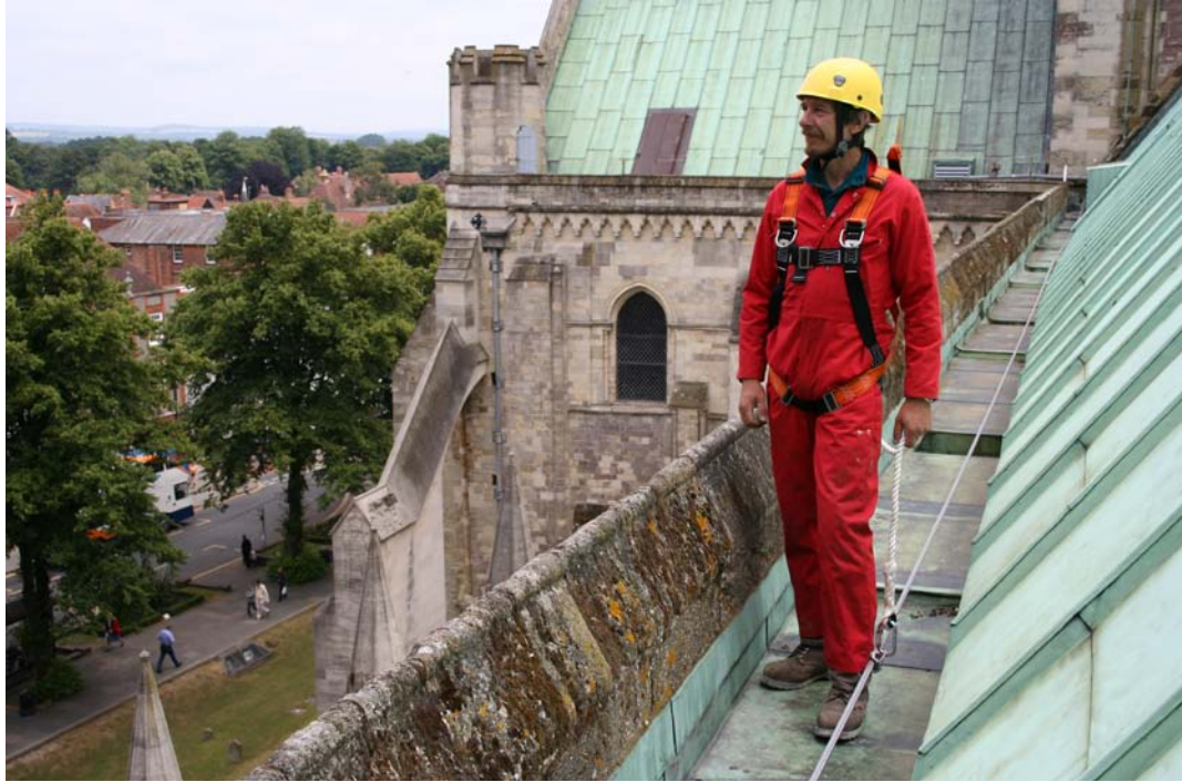
Grey coloured Uni16 synthetic lifeline fitted to the Nave roof, Chichester Cathedral.
