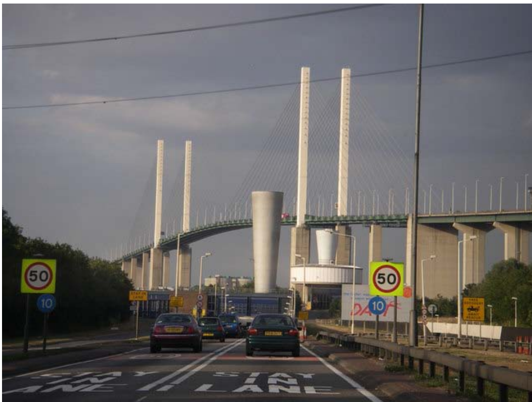
The conical Kent side ventilation stack
