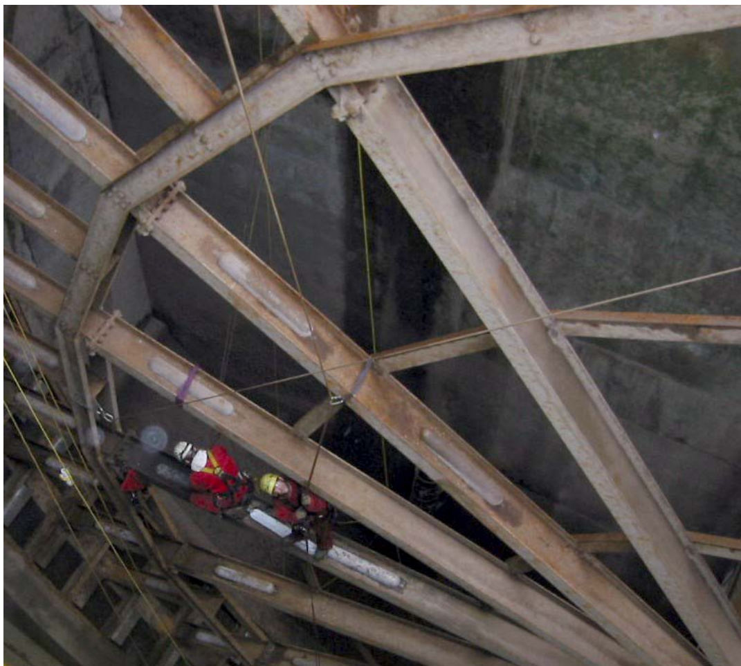
Installation of anodes.
