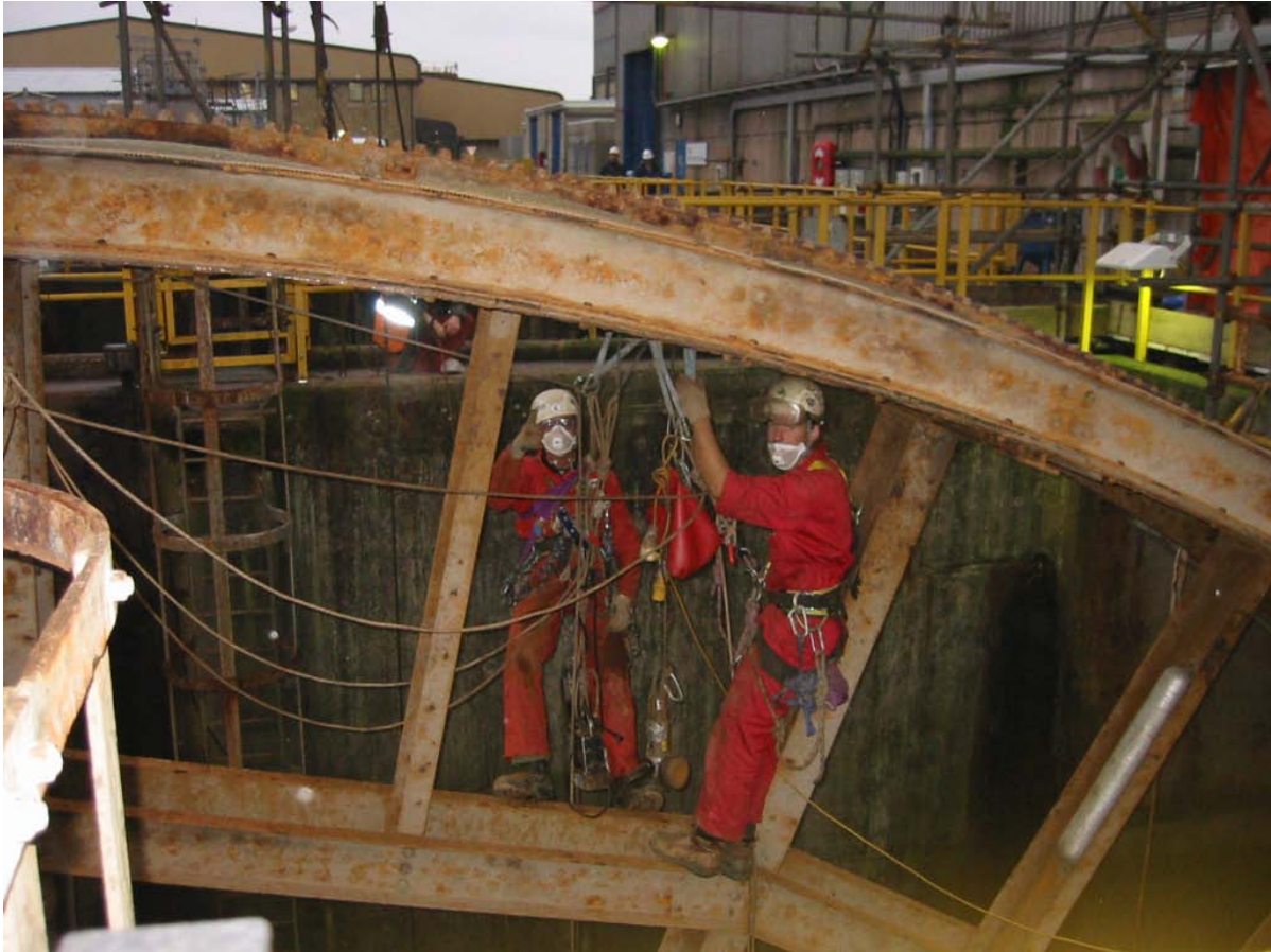
The last anode installed.
