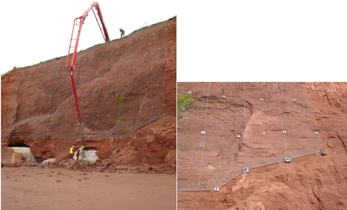
Pumping concrete into caves and Rock netting detail
