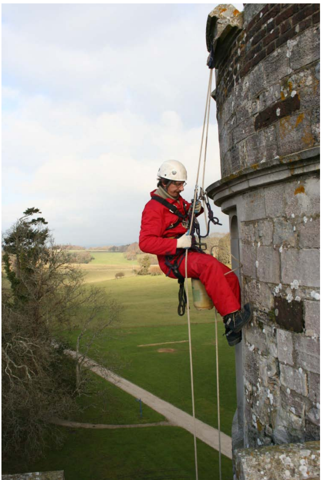
Vegetation removal and weeding
