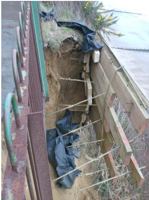
The collapsed cliff top and failed old timber revetment
