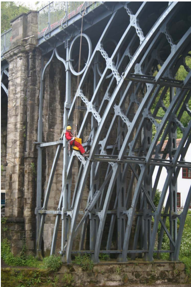
Hands on inspection of the bridge
