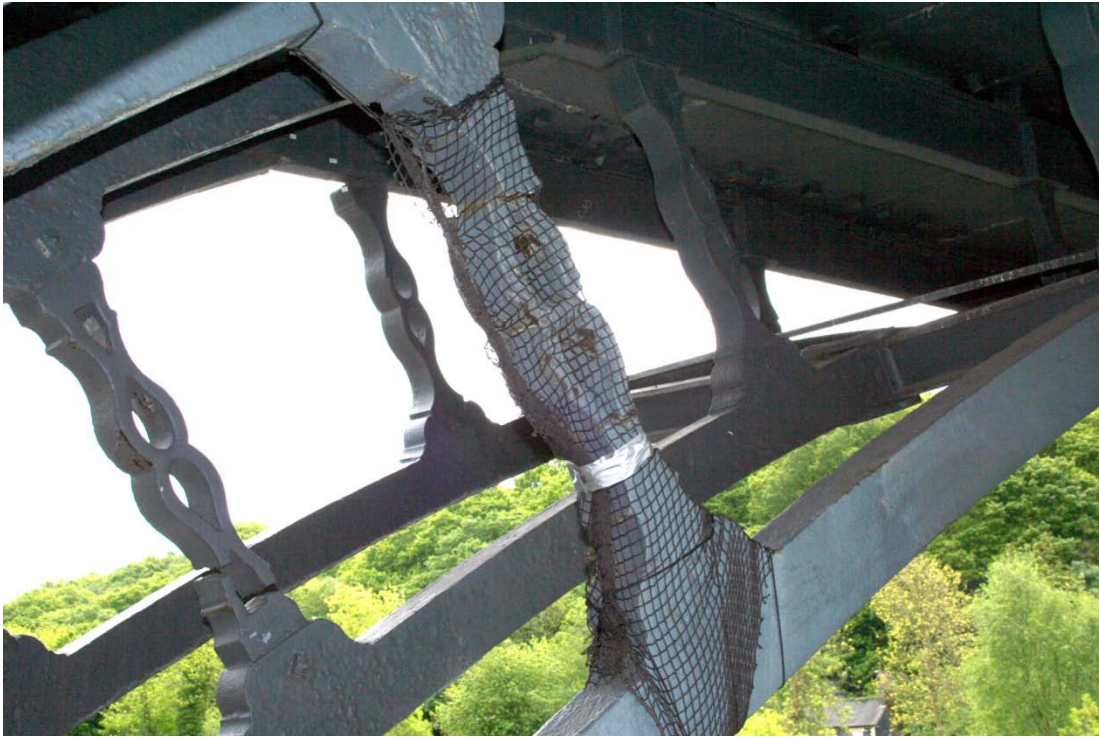
Safety netting around the iron lattice
