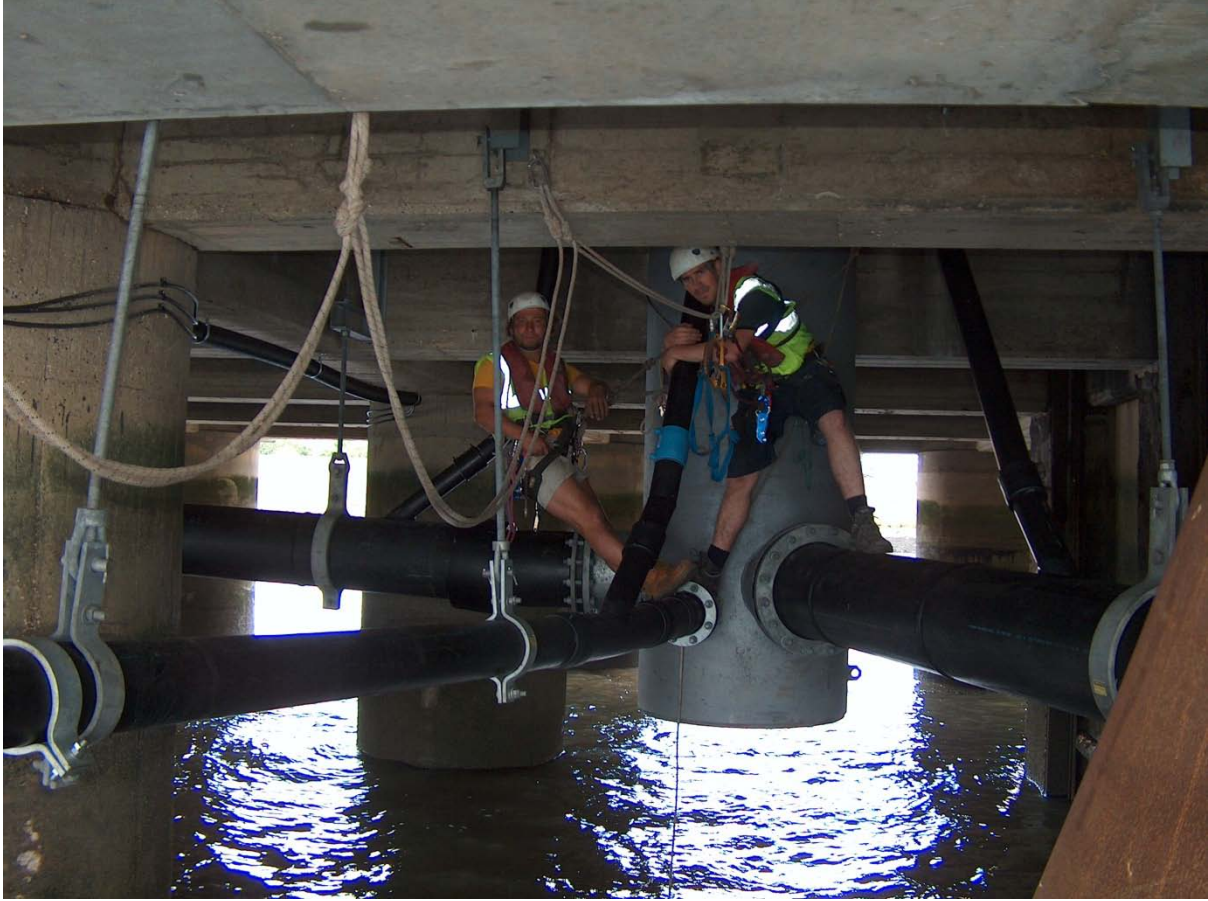
The most complicated section around a sump completed
