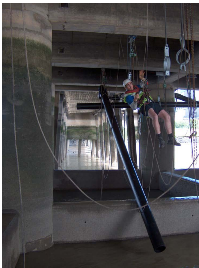
Materials are brought in at high tide and fitted during low tide
