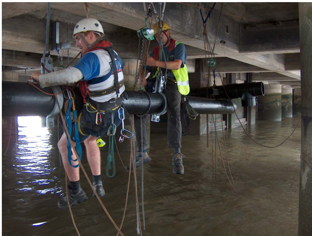
Component parts are lifted into position
